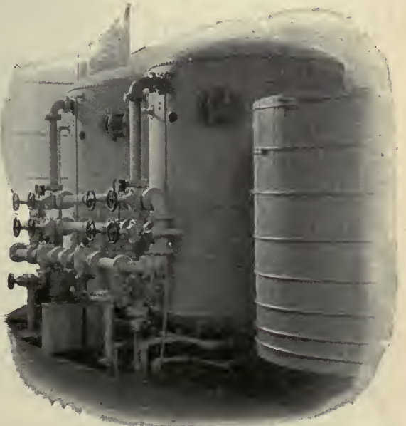
TYPICAL 24-HOUR BOILER FEED-WATER SOFTENING PLANT
